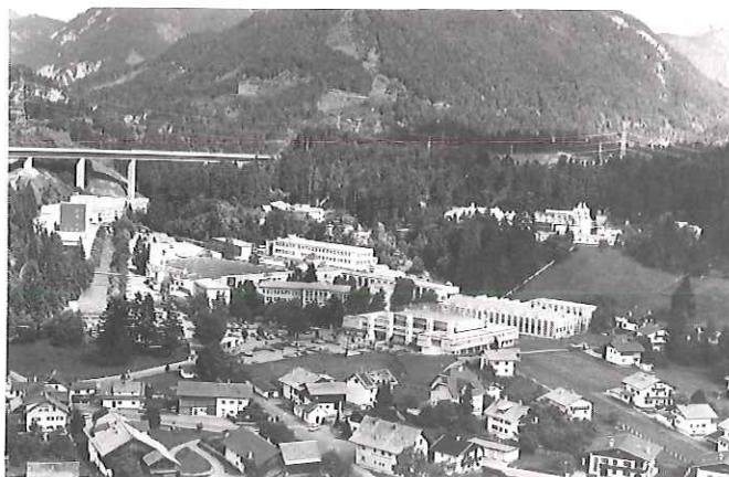
Metallwerk Plansee at Reutte, Austria.
