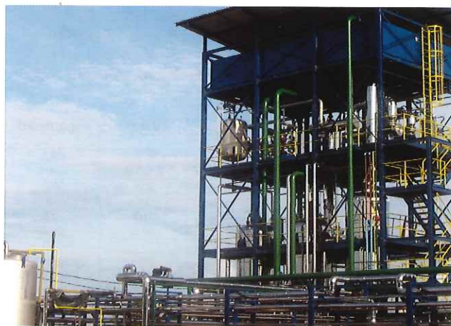
Figure 7: Industrial plant for the production of biodiesel from the esterification of free fatty acids of palm oil operated by AGROPALMA (Belém, PA Brazil). (Courtesy: AGROPALMA GROUP)
